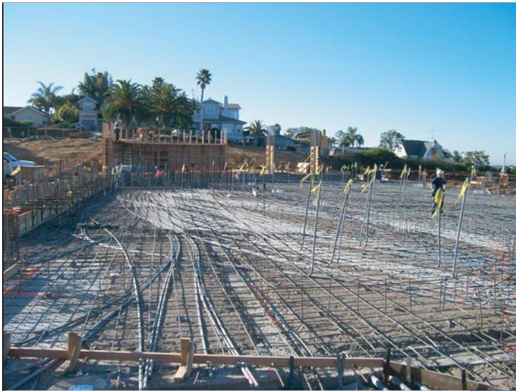
Foundation ready to be poured!
