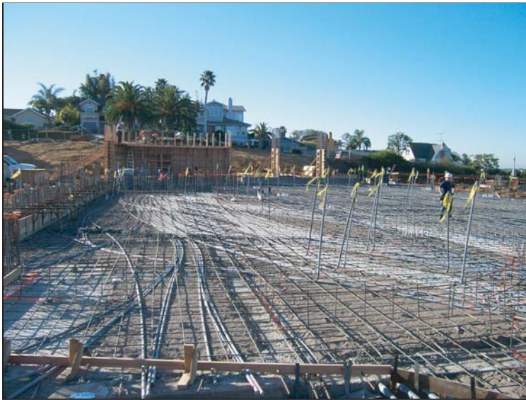
Foundation ready to be poured!
