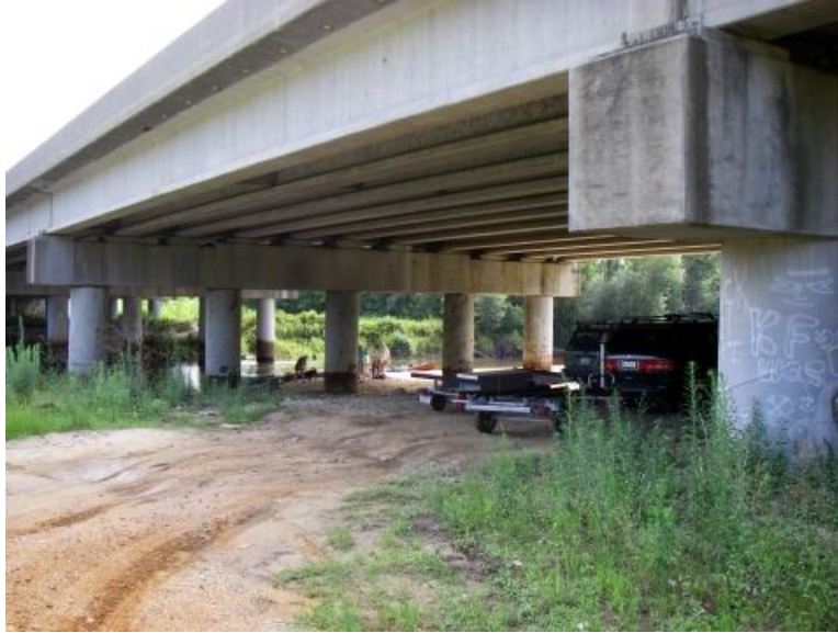
US 29/US 31 Bridge in Flomaton, AL
