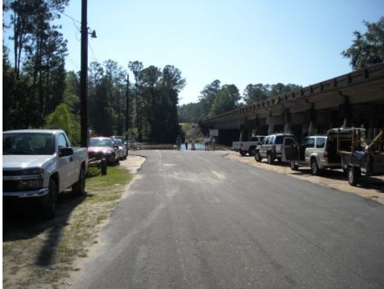
Hwy 90 Shoal River Bridge
