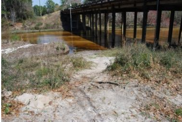
CR-285 Shoal River Bridge
